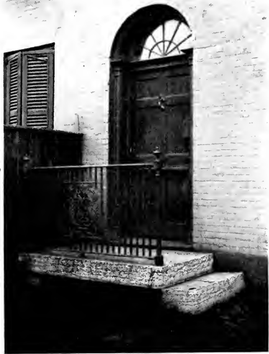
One of the Entrances to the Residence of Hon. A. A. Yates, on Washington Avenue.
